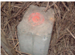
MTO Concrete Monument
